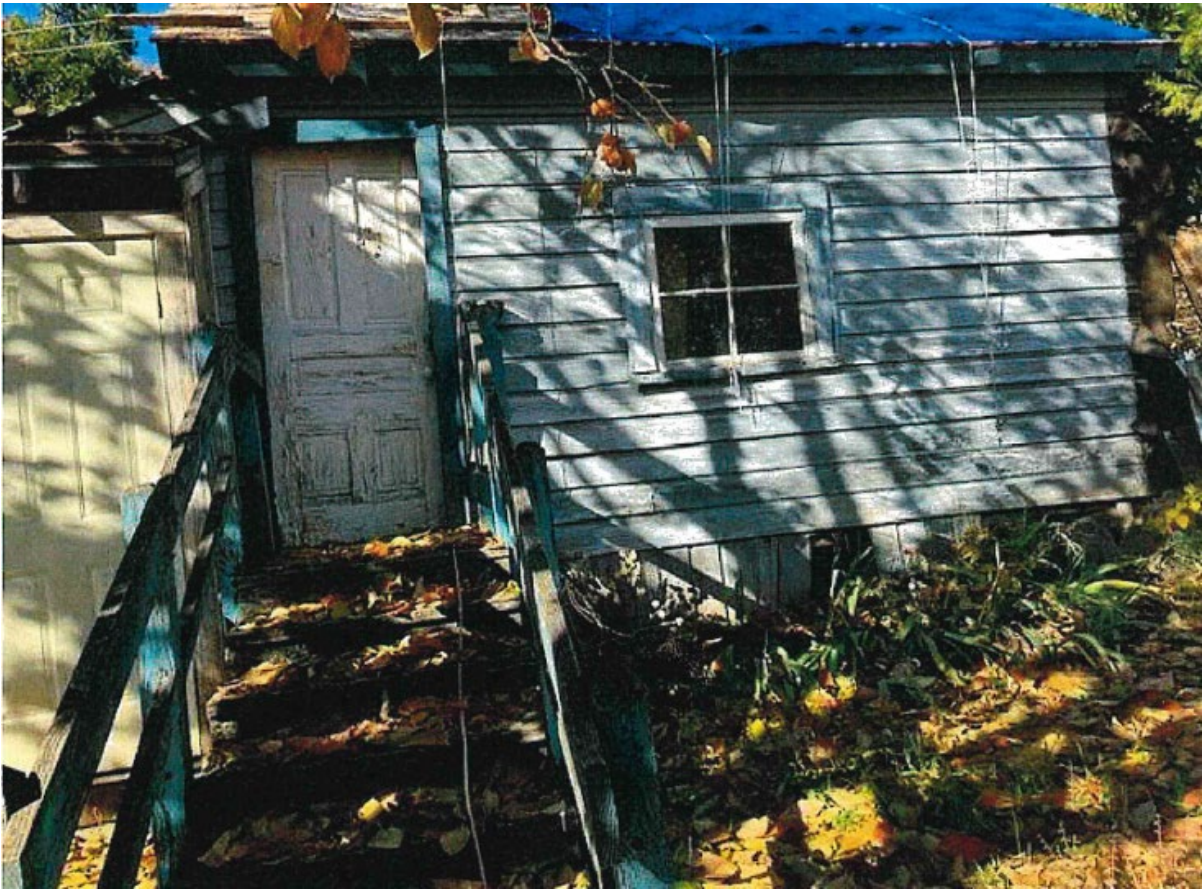
Figure 2-B. Detached Garage - View from back yard facing east.
