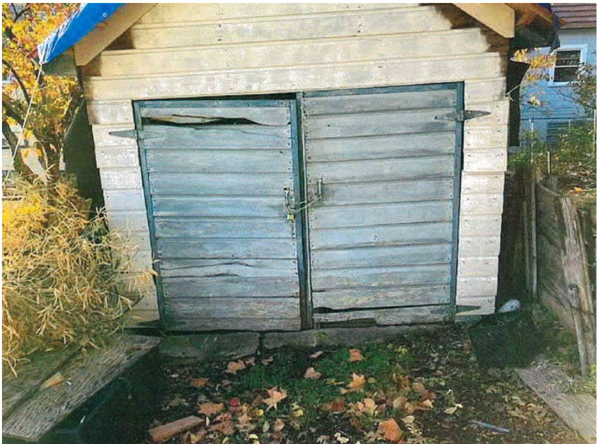
Figure 2-A. Detached Garage - View from Spruce Street facing south.
